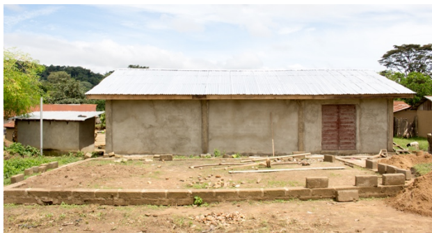
The storage facility and dry floor during construction
