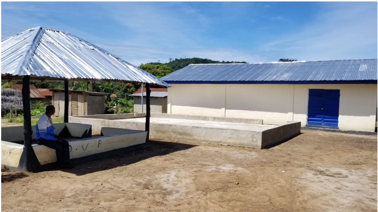
The completed storage facility and dry floor in Pejewa
